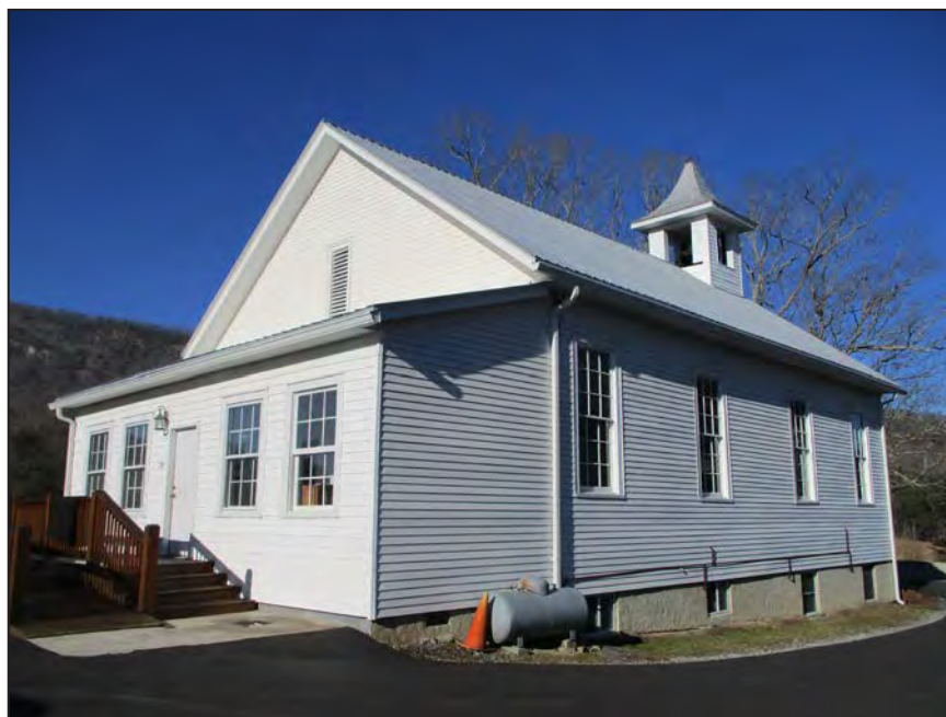
Photograph 7: Oblique view of Tuckasegee Wesleyan Church; looking west. (2018)
