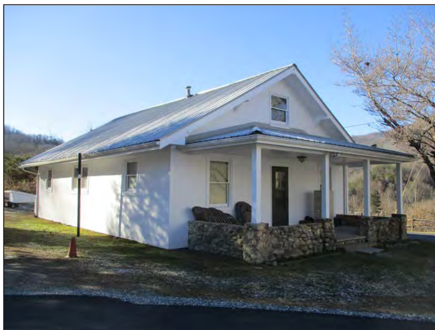
Photograph 10: Oblique view of Tuckasegee Wesleyan Church Parsonage; looking southwest. (2018)
