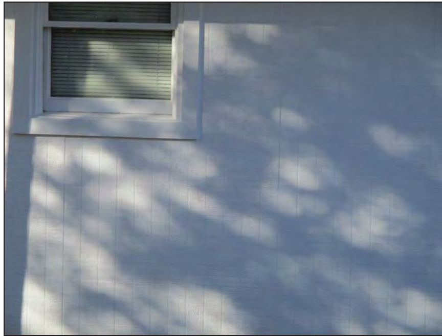
Photograph 11: Detail view of T1-11 siding on Tuckasegee Wesleyan Church parsonage; looking west. (2018)
