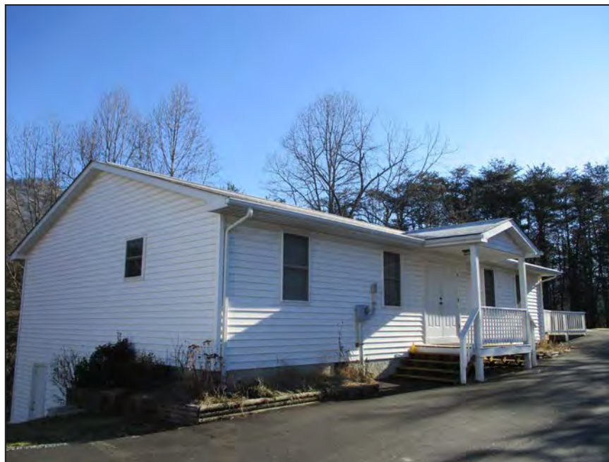
Photograph 12: Oblique view of Tuckasegee Wesleyan Church's Fellowship Hall; looking east. (2018)
