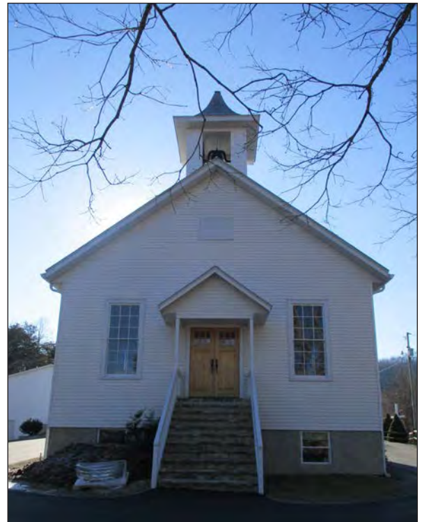
Photograph 1: Façade Tuckasegee Wesleyan church looking southeast. (2018)
